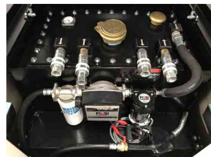
Diesel transfer pump setup
